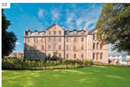
01 Cholsey Meadows in Oxfordshire 02 Royal Barham House in Truro, Cornwall 03 Riverside in Godalming, Surrey
