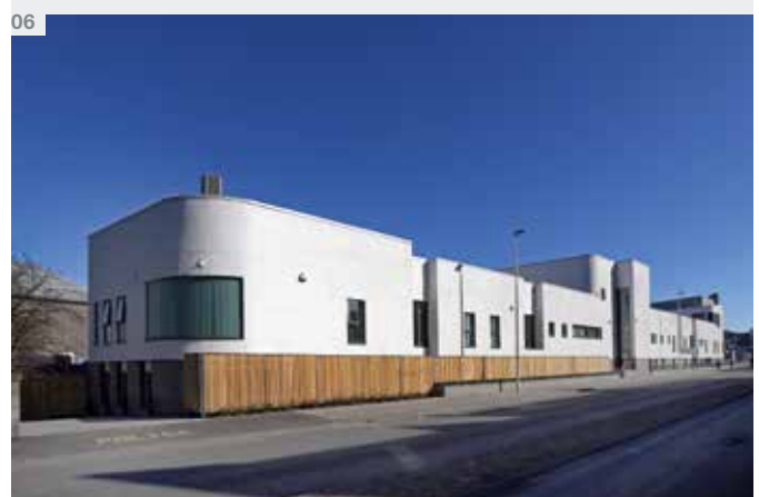
04 Express Park, Bridgwater, part of the Avon & Somerset PFI Scheme 05 James Gillespie's High School in Edinburgh 06 Aberdeen Community Health and Care Village
